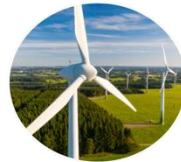
Windmill maintenance Energy and utilities
